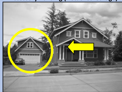
Accessory Building (Detached Garage)
